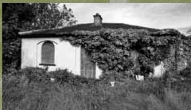
When the Portarlington Ring Road was constructed in 1970, the stretch of the canal that included the second lock was filled in. Today the lock keeper's house stands empty. All that remains of the lock is a portion of the north-west side wall, which is visible from the road.
