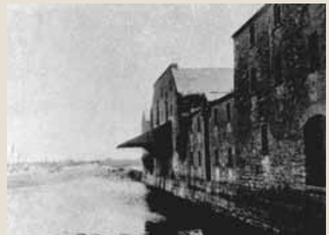
The terminus at Mountmellick had a full harbour, as well as the goods stores shown here.
