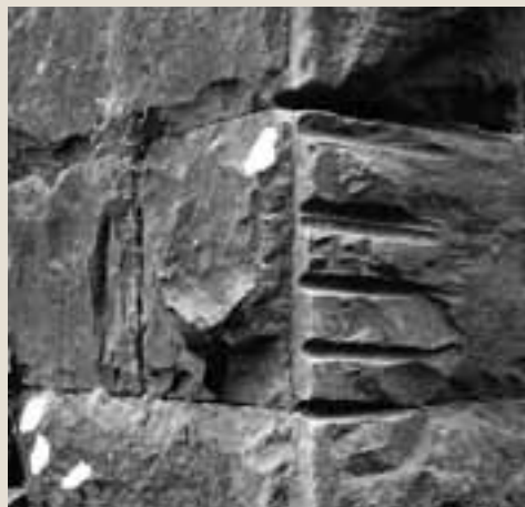
These grooves on the quoin of a bridge were worn by towropes as horses pulled canal barges.
