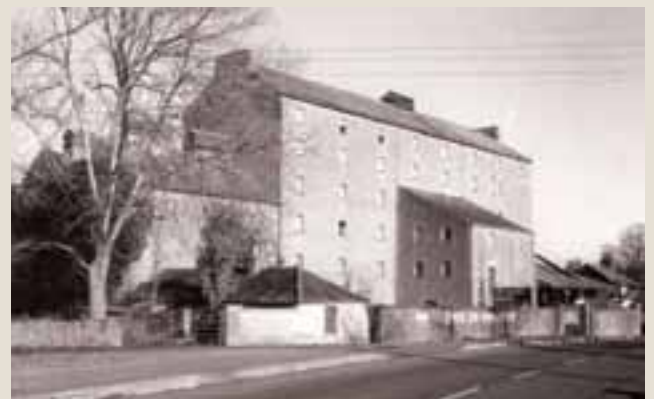
This building was originally a steam-operated flour mill erected in 1840 by Samuel Sheane. In the 1880s, when Eugene Codd took over Irishtown Maltings from James Sheane, he changed the defunct flour mill into a malt house. Codd's shipped its last load of malt on the Mountmellick Canal in 1940. Today the old mill has been converted into the Mountmellick Development Association building.
