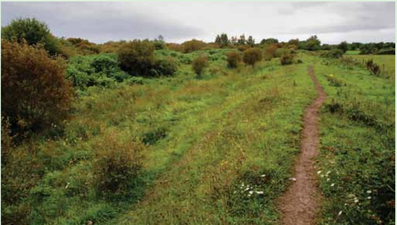
Looking north-west along the dry canal bed just north of the first lock.
