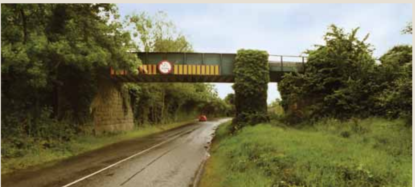
This bridge carried the Dublin to Portarlinton train over the Mountmellick Canal. Today the canal's bed has been filled in to make a road. However, it is still possible to see marks left by barge towropes on one of the bridge's piers.
