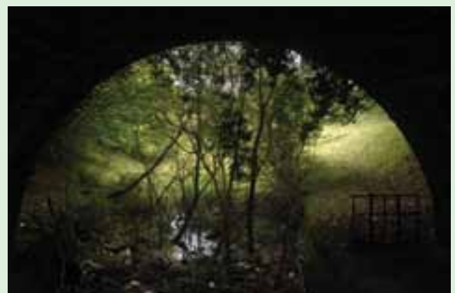
View from beneath Dangan's Bridge
