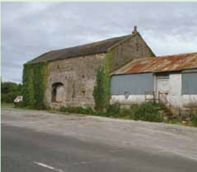
Canal stores along the Mountmellick Canal, now the Portarlinton Ring Road.
